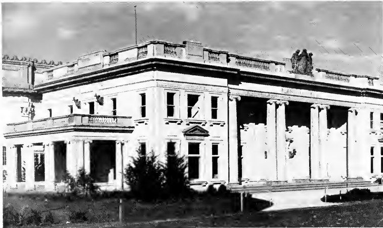
THE WISCONSIN BUILDING
